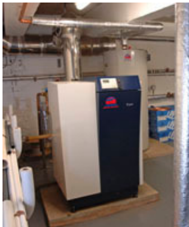
The Supa-Flo high efficiency gas-fired water heater from Andrews Water Heaters
