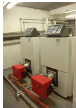
Two NXR3 cast iron sectional boilers from Potterton Commercial
