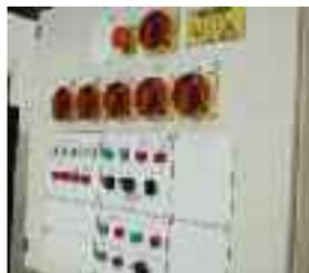
The 0 – 10V signal from either of the methods above, is fed in to a robust and reliable Mitsubishi PLC which controls the system by sequencing and modulating the boilers to closely match the system demand whilst ensuring the system operates at its most efficient by utilising the various heat sources in the correct sequence.
